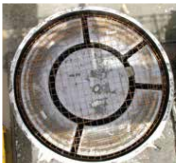
Inverted Mould with Reinforcing Ready for Concrete
