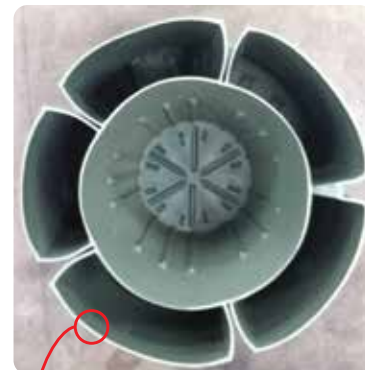
Sectional view of plastic tank internal showing one-piece construction.
